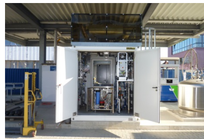
Co-production of H 2 , O 2 , heat @ H 2 fuelling station HyCentA, Graz
